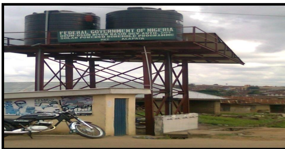
Plate 1: Public borehole located at OkeAlapata, Ogbomoso
